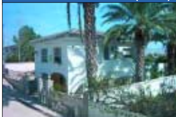
Town House: Baños de Fortuna (Ref 432)
